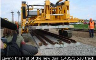
Laying the first of the new dual 1,435/1,520 track sections on the "Rail Baltica" line at Sestokai, Lithuania
